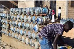
Construction of the school wall with ecobrics (bottles filled with solid waste). Credit: CRES
