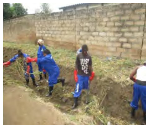
Construction of the drainage. Pictures provided by: People's Process on Housing and Poverty in Zambia
