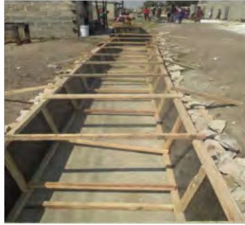
Excavation and concrete lining of the drainage (Photos provided by: People's Process on Housing and Poverty in Zambia)
