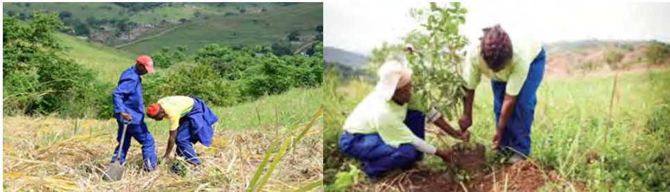
Workers prepare a site for the planting of trees at the Buffelsdraai Community Reforestation Site (Photo provided by Ethekewini Municipality)
