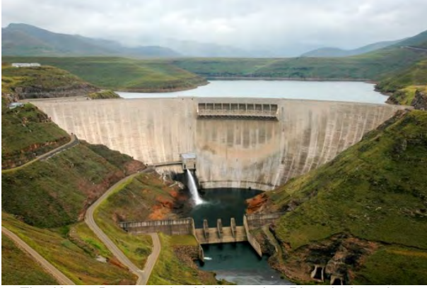
The Katse Dam, on the Malibamat'so River in Lesotho, was completed in 2009, as the centrepiece of the Phase 1 of the LHWP. Photo provided by: Amada44 / Wikimedia Commons
