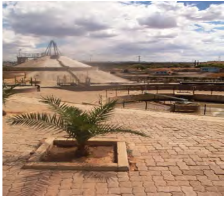
Bioreactor at Gammams water reclamation Plant. Photo provided by: City of Windhoek
