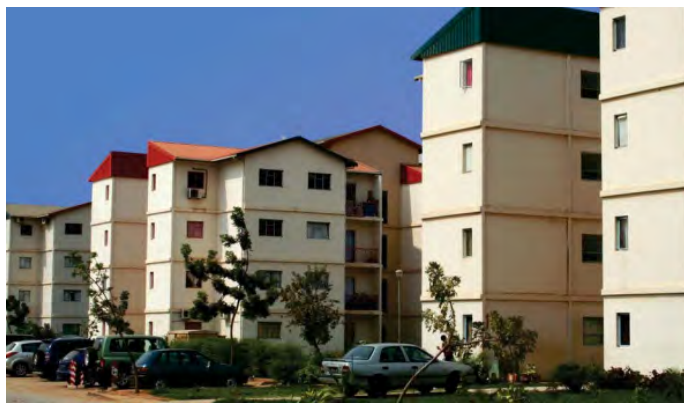
Nova Vida Housing Development Photo provided by: Aurecon
