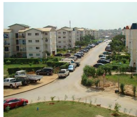
Constructed part of the Park. Photo provided by: Aurecon
