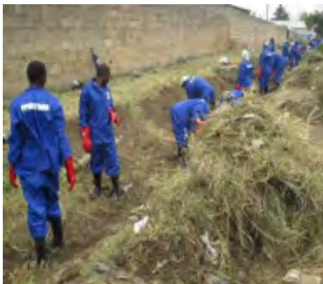
Community volunteers working on the drainage. Pictures provided by: People's Process on Housing and Poverty in Zambia
