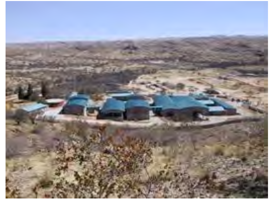
The Water Reclamation Plant in Windhoek is internationally known as the first plant in the world to reclaim domestic sewage for potable use. Photo provided by: City of Windhoek
