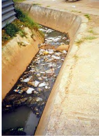
Waste in the drains of Lusaka. Picture provided by: Lusaka Times
