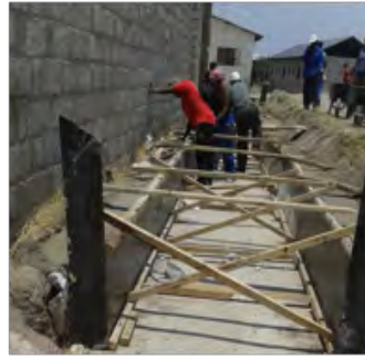
Excavation and concrete lining of the drainage (Photos provided by: People's Process on Housing and Poverty in Zambia)
