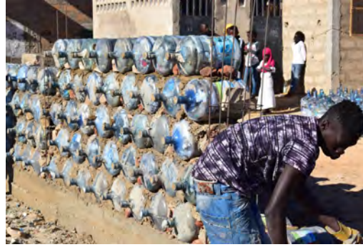
Construction of the school wall with ecobricks (bottles filled with solid waste). Credit: CRES
