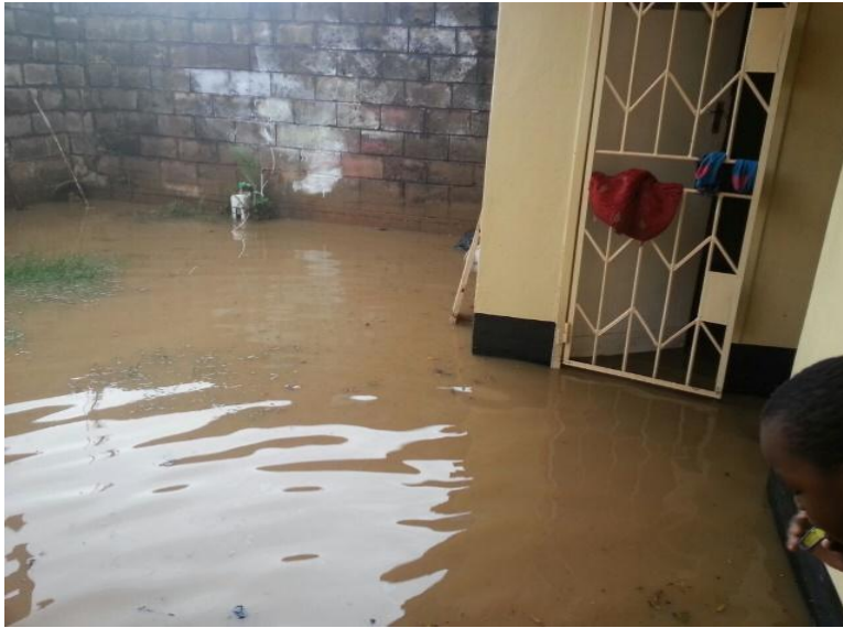
Figure 1 A flooded house in Kabwata, Lusaka
