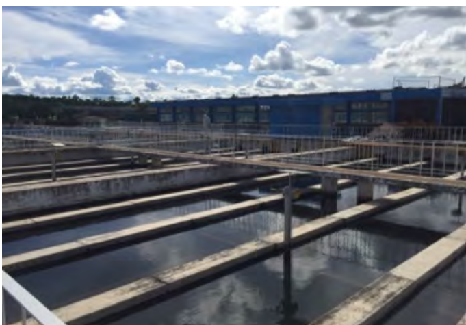
Figure 3 | Iolanda water treatment works Lusaka Zambia
