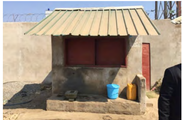
Figure 4 | Water kiosk in Kanyama peri-urban area
